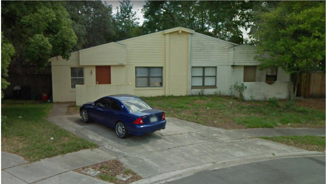
Facing south towards front of subject property, the subject residence is on left
