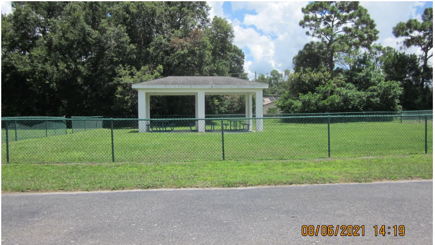
Unpermitted gazebo facing east
