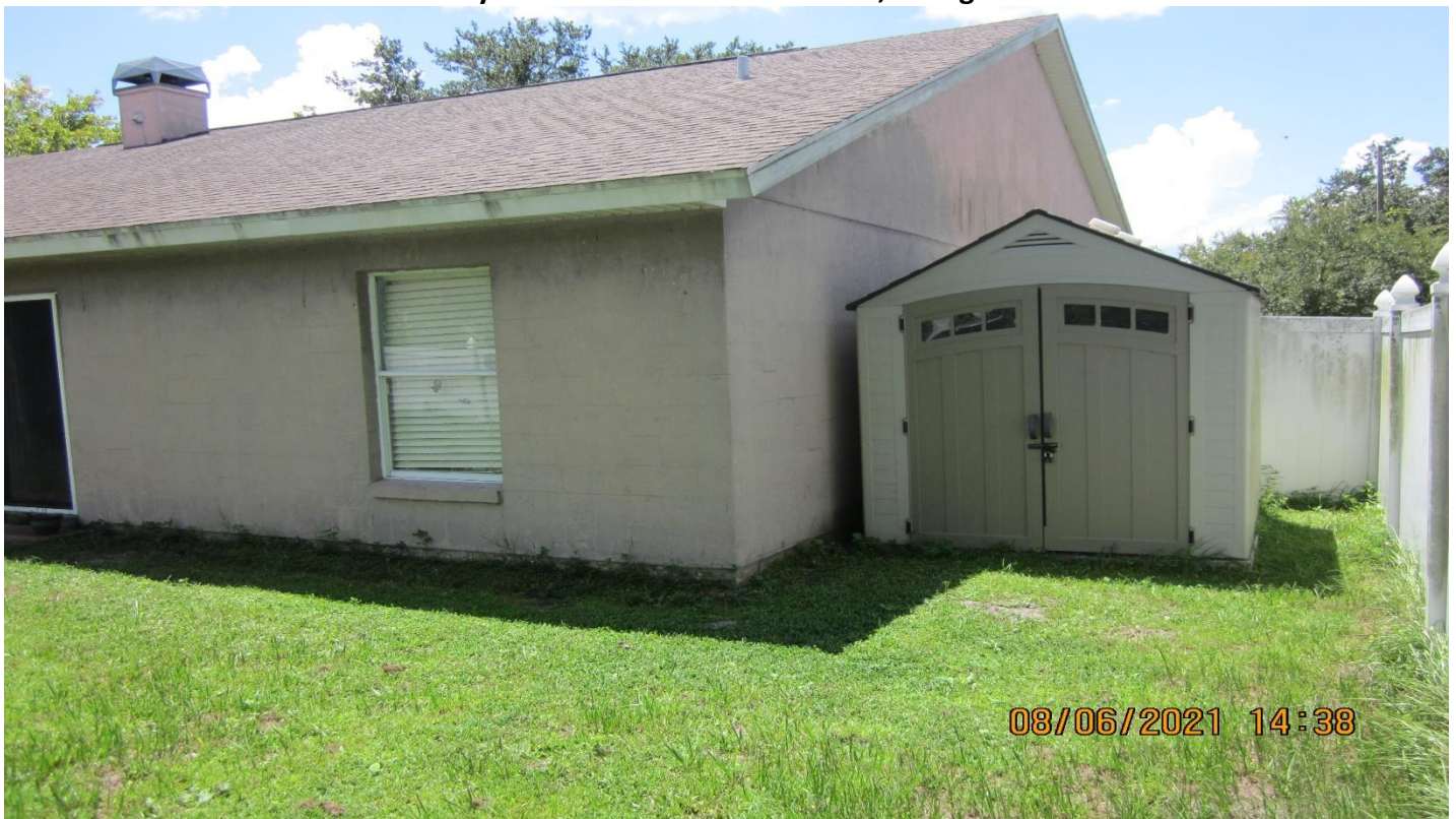
Unpermitted shed to be removed facing west
