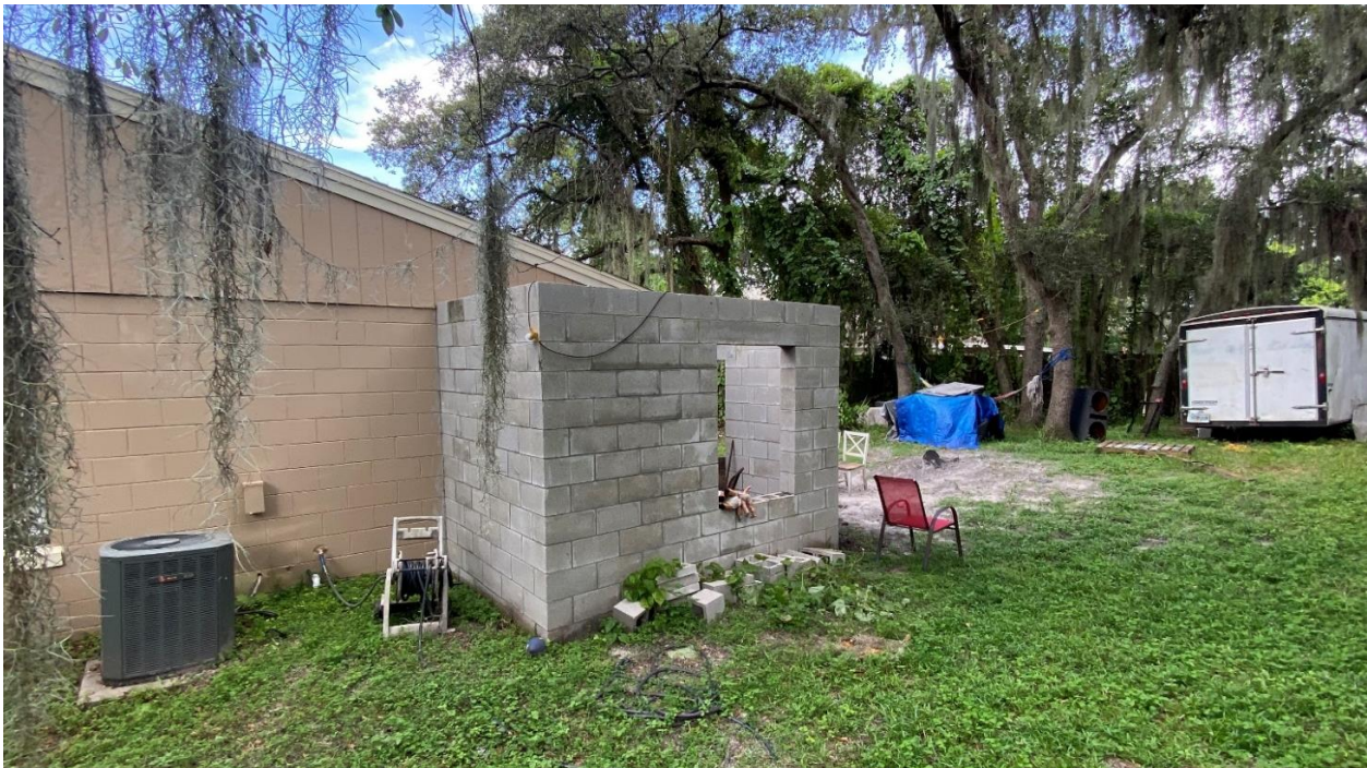
Rear yard, facing northeast towards addition
