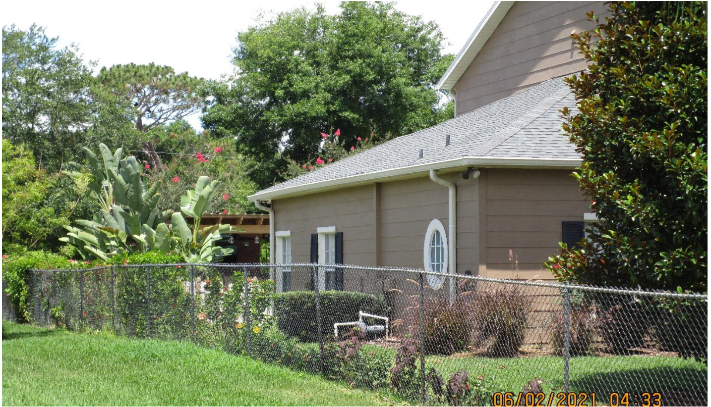
Unpermitted covered deck/gazebo behind house
