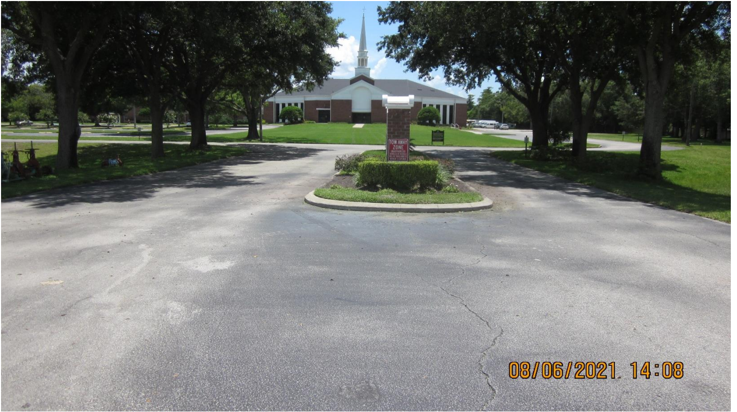
Front from Lake Underhill Rd.
