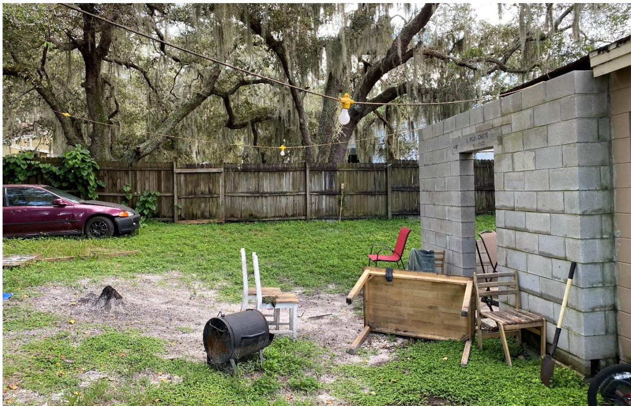
Facing south towards rear of property (addition is to right)
