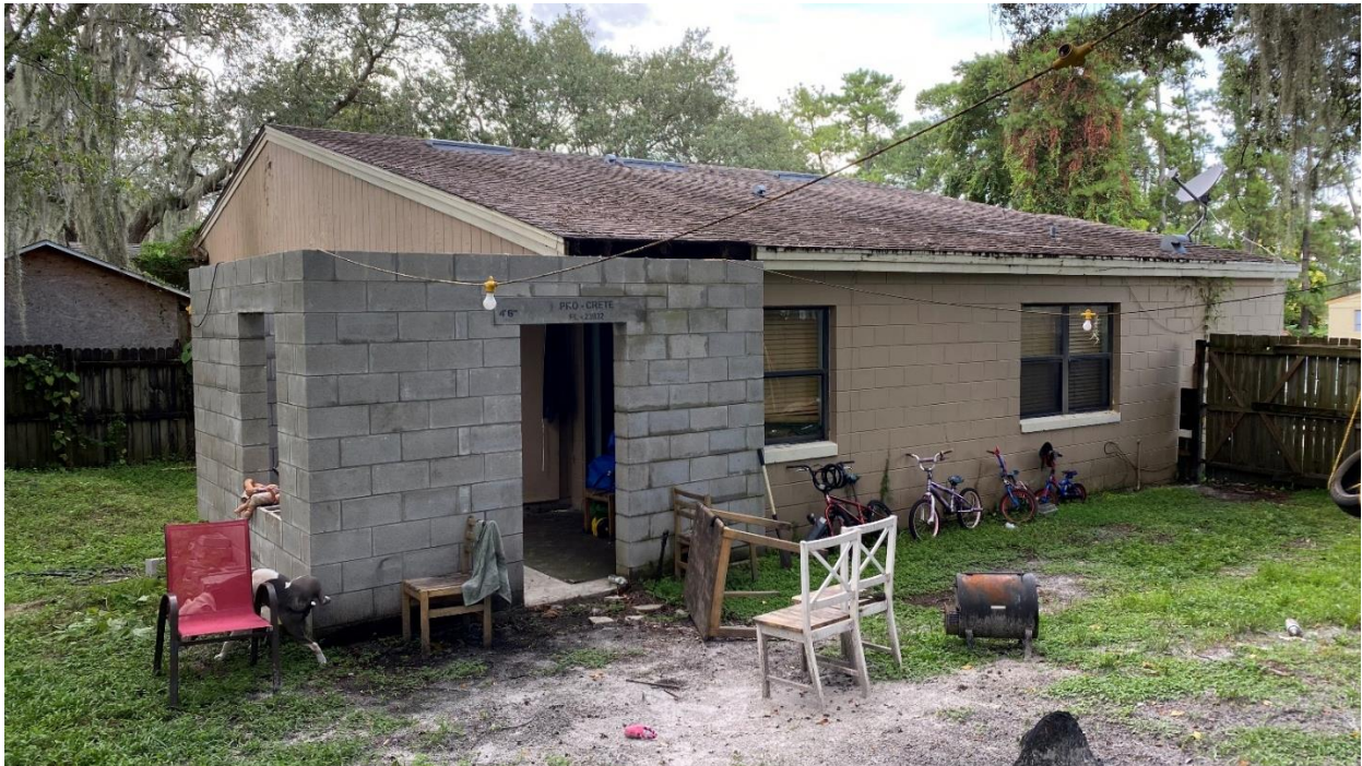
Facing northwest towards front of property and adjoining duplex
