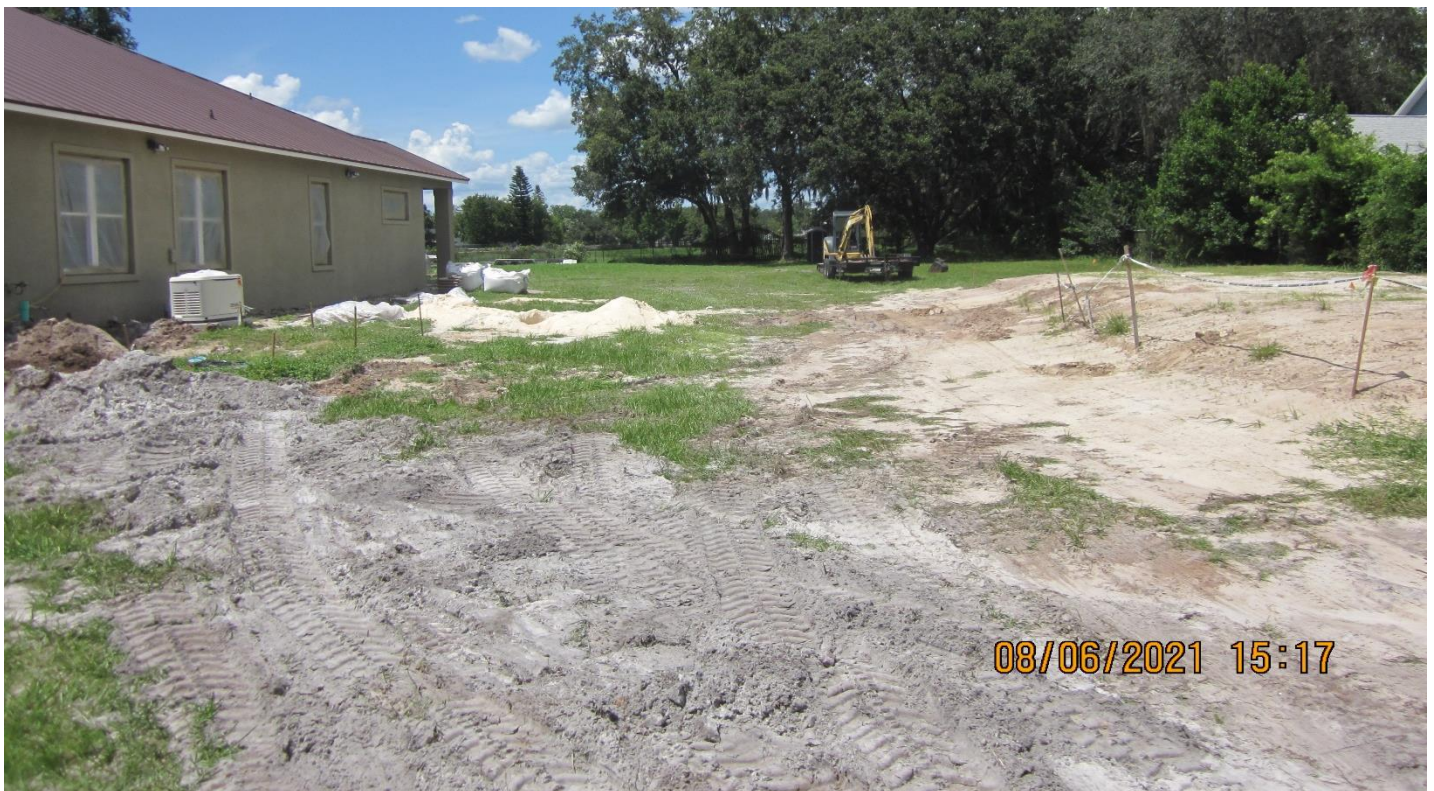
Proposed accessory structure location facing north
